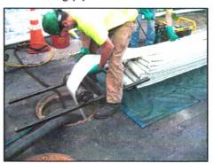
The project included relining over 13,000 LF of existing sewer line, replacement and/or rehabilitation of approximately 80 manholes, and rehabilitation of the 13<sup>th</sup> Street pump station.
