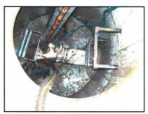
smoke testing, manhole inspections, and evaluation of problem areas. Upon review of the inspection and subsequent report performed and provided by Triad, it was decided that it was more economical to slip line the existing pipe and to rehabilitate the existing manholes.
